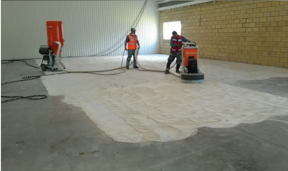
Concrete Grinding Effect
