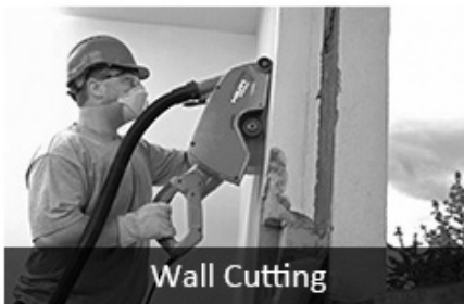
Concrete With Rebar Cutting
