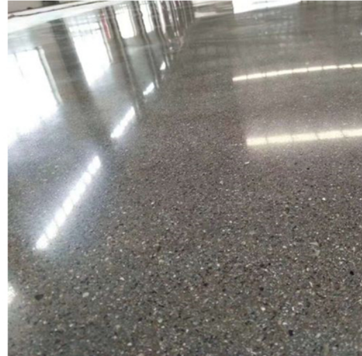
After Grinding and Polishing
