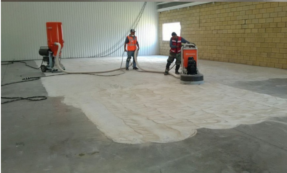
Concrete Grinding Effect
