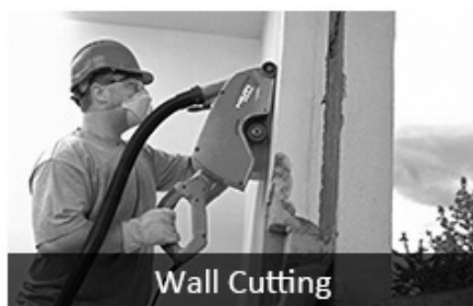
Concrete With Rebar Cutting
