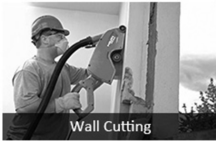
Concrete With Rebar Cutting
